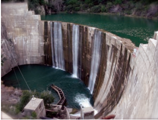
Removal of Matilija Dam would improve habitat for endangered southern steelhead. Photo by Jacob Katz.
