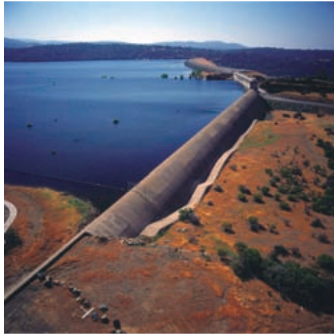
Better integration between water supply and flood management of reservoirs will become increasingly important. Photo by California Department of Water Resources.
